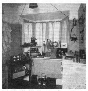
Another old timer outfit—G2NS in 1933. He ran a crystal-controlled SP5SR-SP5SR-LS5B transmitter, with an AR4100-PT25 modulator; the receiver was the ubiquitous 1-V-1, using PM12-HL210-PM22.
