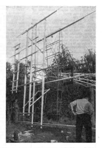
Not a disaster, nor yet a radar aerial array, but the top of VK3KU's composite votary beam for 14, 28, 50 and 166 mc, lowered for inspection.
