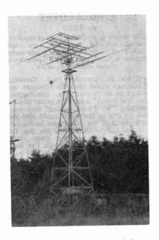
VK3KU's beam system in position. It weighs four tons and the mast itself is insulated from ground, enabling the whole assembly to be operated as a capacity loaded quarter-wave vertical aerial for 7 mc!
