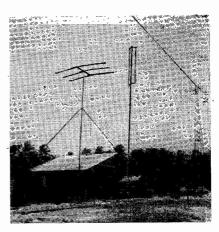
General view of G6CU/ZC2, the famous station on Cocos Is. The 3-element rotary is beside the hut, and the 105 ft. tower in the background carried the Sterba array, put up latterly.
