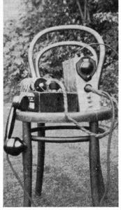
The portable equipment used by E12J in the September 56 Mc Tests. He worked GW6AAP, at 112 miles with one watt input.
