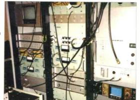
A rack containing intermediate amplifiers and filtering for the Mk2 radio telescope as well as frequency distribution to Jodrell Bank's remote telescopes from the Atomic Standard Frequency.
