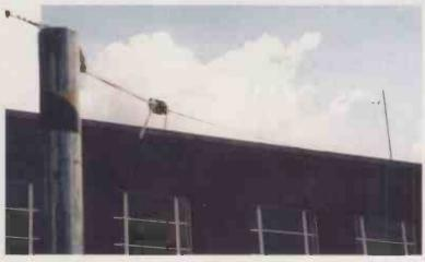
The 'bottom end' of the inverted L antenna looking onto the metal-skinned roof area.
