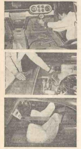
Top. Final fitting of the steering column to a Falcon GT, It comes with the body and chassis pre-assembled. Centre. The engine requires fitting in the Falcon but the wiring loom is in place, ready to connect.
