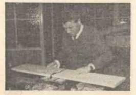
Fig. I.—Cross-cutting the plank into 10½-inch lengths. Apply even pressure to avoid pinching saw.
