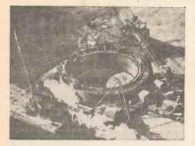
This is a circular steel caisson sinking down into the mud beneath the waters of the Stralts of Mackinac in the United States. Barge mounted cranes dig out the mud from inside the caisson whilst the sides are slowly built up.
