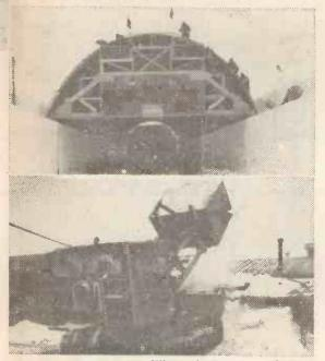
D-4 Traxcavator filling the snow melter at McMurdo Sound base.
