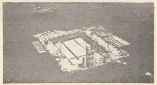
A temporary wall has been built around the site of this bridge foundation, the water pumped out and the cutting edge of the rectangular box caisson assembled on the dry floor. Slowly it will sink down through the mud, the sides being added to all the time, to keep them above the surface.
