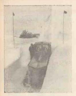
The first step in the preparation of a city under the ice. A snowmiller cutting one of the many trenches of New Byrd.
