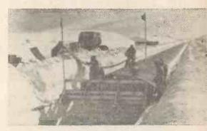
The second step . . . Installing archways in the excavated trenches.
