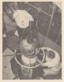
The Vanguard satellite is installed atop the satellite launching Vehicle 7 at Cape Canaveral.
