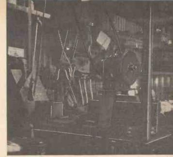
This is a view of a grinder showing drive from overhead countershaft.
