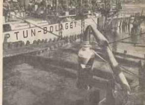
Fig. 6.—One of the Flygt submersible pumps being lowered into place.
