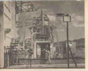
A close-up of the U.S. Atomic Energy Commission's "Kiwi-A-Prime" nuclear reactor, the Commission's second reactor made to test the feasibility of nuclear propulsion for space vehicles.
