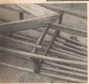
Photo 4.—Close up of the splayed boards.
