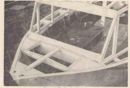
Fig. 23.—The fore deck framing.
