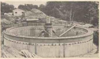
Fig. 3.—The base for a low-noise horn antenna under construction at the satellite communication station site at Holmdel, N.J.
