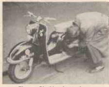
Fig. 2.—Checking the air cleaner.
