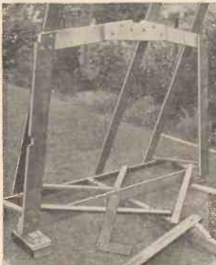
Fig. 1.—Frame 1 braced in position on the building form.
