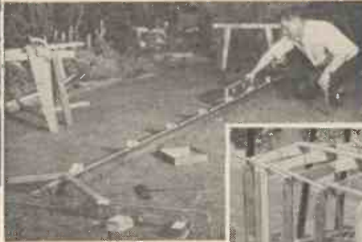
Fig. 6.—Frame assembly temporarily cramped together.
