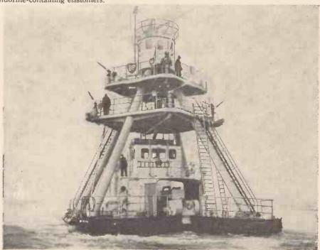
The photograph above shows the Swansea Docks firefighting craft, "The Firemaster." Built catamaran style, it has an open tower with nine fire-fighting nozzles operating from three decks. It is possible to pour 4,000 gallons of water or 12,500 gallons of foam a minute on to a fire. Operations are controlled from the top of the 40ft. tower.
