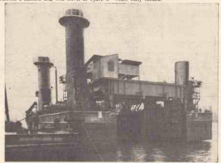
The second mobile oil drilling platform to be constructed in the United Kingdom has been built at Wallsend-on-Tyne. The £500,000 Triton contains 1,500 tons of steel, has been built for operations in water depths up to 120ft. and is fitted with four retractable legs, each of 200ft. in length and 8ft. in diameter.
