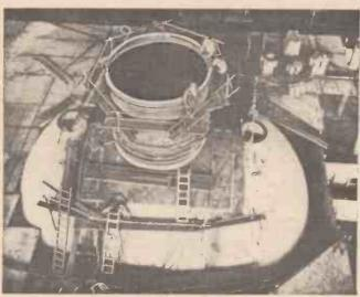
Fig. 6.—The top of the reactor pressure vessel for N.S. Savannah in position.
