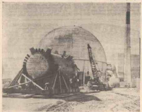
The 350-ton atomic reactor for the power station before it was moved into the 190 ft. steel sphere shown in the background.
