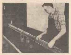
(Above) A bundle of 10ft. long fuel rods is assembled to make one of the 488 fuel elements.
