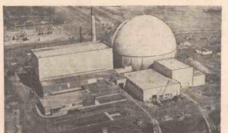
adjacent to the sphere houses the turbinegenerator and other equipment necessary for converting the thermal energy of steam into electrical energy.
