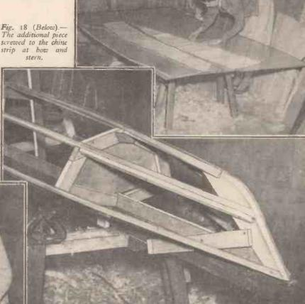
Before fixing the three remaining panels it is as well to fair off the edge of this first panel at the chine stringer so that the builder is better pre-pared for the task on the other three. From Fig. 20, it will be observed that the plywood has to be filed away to a very oblique angle towards the bow. Many of the nails will be found to be in the way. They must be punched down because they would catch in the treth of the file and be dragged sideways in the plywood. When doing this
