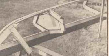
Fig. 12 (Above).-Frames in place and keelson fitted.
