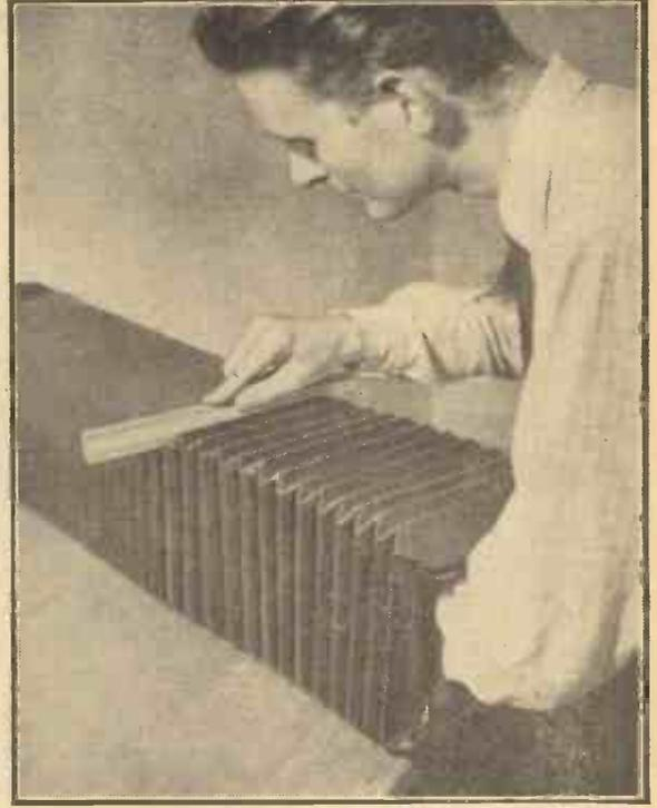
Fig. 6 (Right).—Inside folds being made with the aid of a rule.
