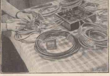
Fig. 7.—Testing one of the junction boxes with a battery and bulb.
