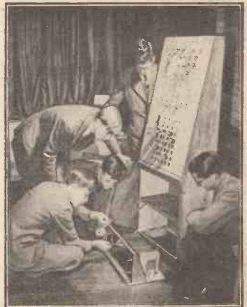
The photograph shows some of the boys who built the computer, also the machine itself. A fuse is being replaced in the power pack by one of the younger boys.
