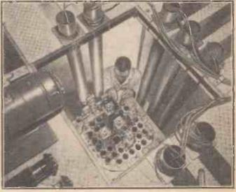
Fig. 1 .- A technician adjusts a control rod in the core of a nuclear power plant.
