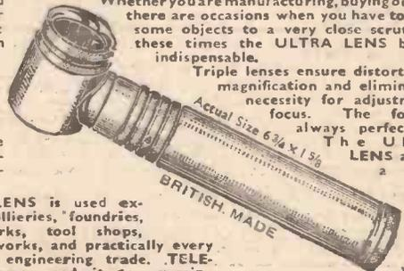
Triple lenses ensure distortion-free magnification and eliminate the necessity for adjustment of focus. The focus is always perfect.
