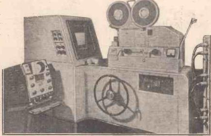
General view of one of the 35 mm. suppressed frame television recording assemblies showing part of the picture display tube and the monitoring oscilloscope. In front of the main display tube can be seen the pistol grip photometer used for measuring the screen brightness of the display tube. See final paragraph.
