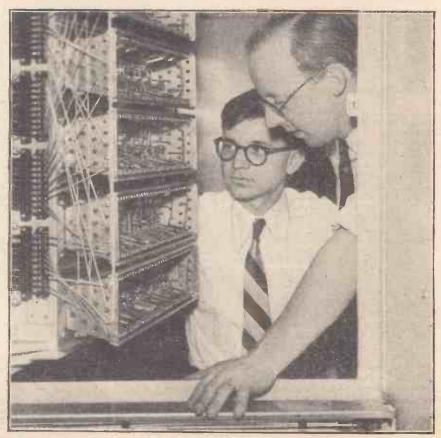
Canada's first mechanical brain is nearing completion at the University of Toronto. with a section representing about one-fiftieth of the thinking robot, is Dr. C. C. Gottlieb (left), director of the University Computation Centre, and Brian Pollard, chief engineer of the computing section of Ferranti's in England from where the machine was brought.
