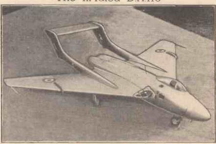
The D.H.110 fighter 'plane, which is powered by two Rolls-Royce Avon jet engines, combines the well known de Havilland twin-boom construction with swept-back wings. It was in this machine that the test pilot, John Derry, lost his life when flying through the sound barrier, at Farnborough, in September.
