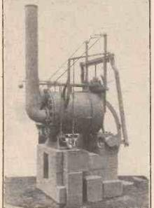
Fig. 1.—Trevithick engine and boiler. The directacting high pressure steam engine, patented by Trevithick in 1802 for stationary and locomotive use, eventually superseded the beam engine. This engine, found at Hereford in 1882, was made about 1805 and probably developed 7 h.p. with steam at 50lb. per sq. in.
