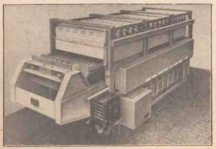
The feed end of an infra-red ore-drying machine, manufactured by the Fraser and Chalmers Engineering Works of the General Electric Company, Ltd.
