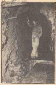
Fig. 2.—One of Mr. Oswald's assistants is seen here in the south-west spiral tunnel on the model railway during the concreting of the floor. The floor has already hardened where he is standing.
