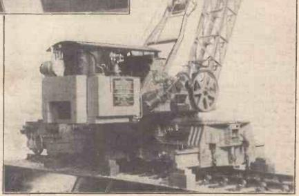
Fig. 1.—This huge working model of a Craven Railway Service Crane is one of the most spectacular built by the late Mr. S. J. Ward. It is to a scale of 1/10th full size.
