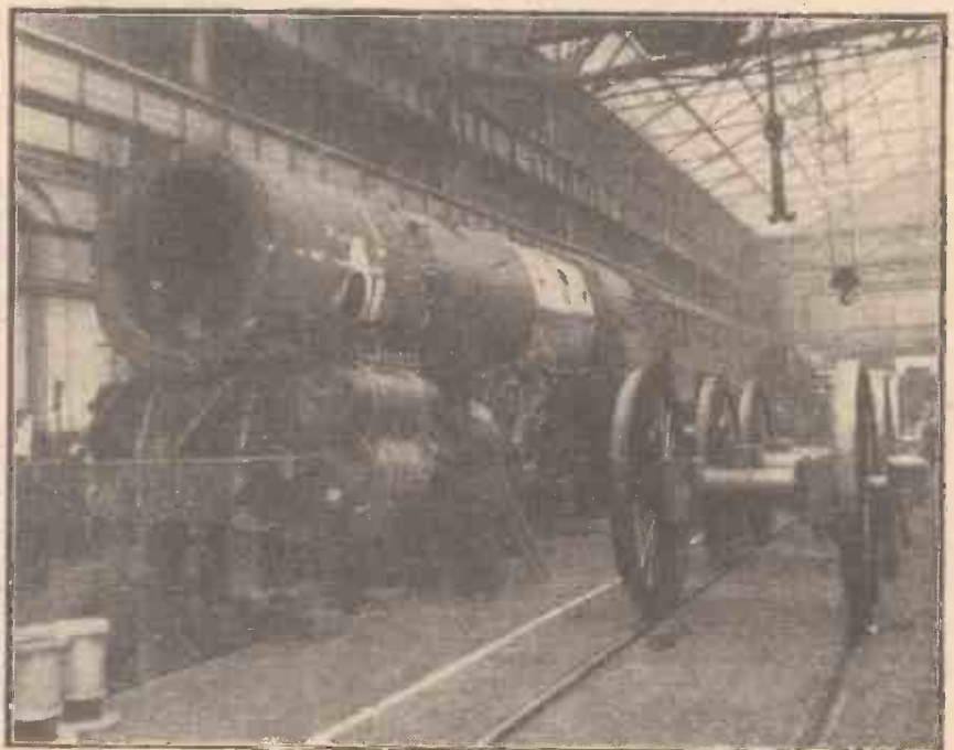
One of the new standard British Railways locomotives being prepared for wheeling in the erecting shop, at Crewe.
