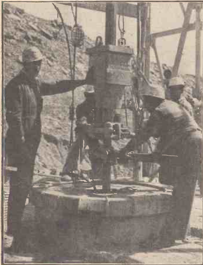
Unscrewing the drillpipe.
