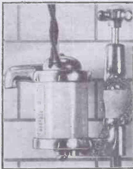
Fig. 22.—Three types of instantaneous water heater. One (a) has an electrical loading of 4 kW. and provides a constant flow of 2½ pints of water per minute with a temperature rise of 70 deg. F. above the incoming water supply, e.g., 45+70=115 deg. F., while (b) is a further type which for bath use has an 8 kW. loading. On the right is a small instantaneous water heater which can be placed on the outlet of an ordinary cold water tap. The local supply authority should be consulted before any of these are installed.
