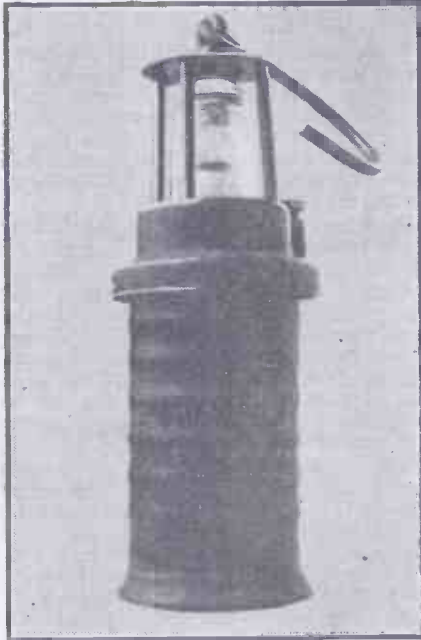
The flame lamp displaced. An early accumulator electric lamp for mine illumination.
