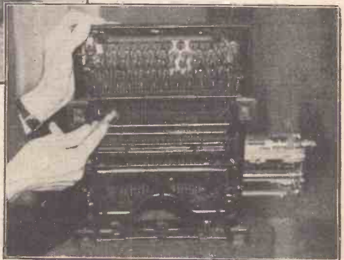
(Above) Cleaning the type with a small brush dipped in methylated spirit.
