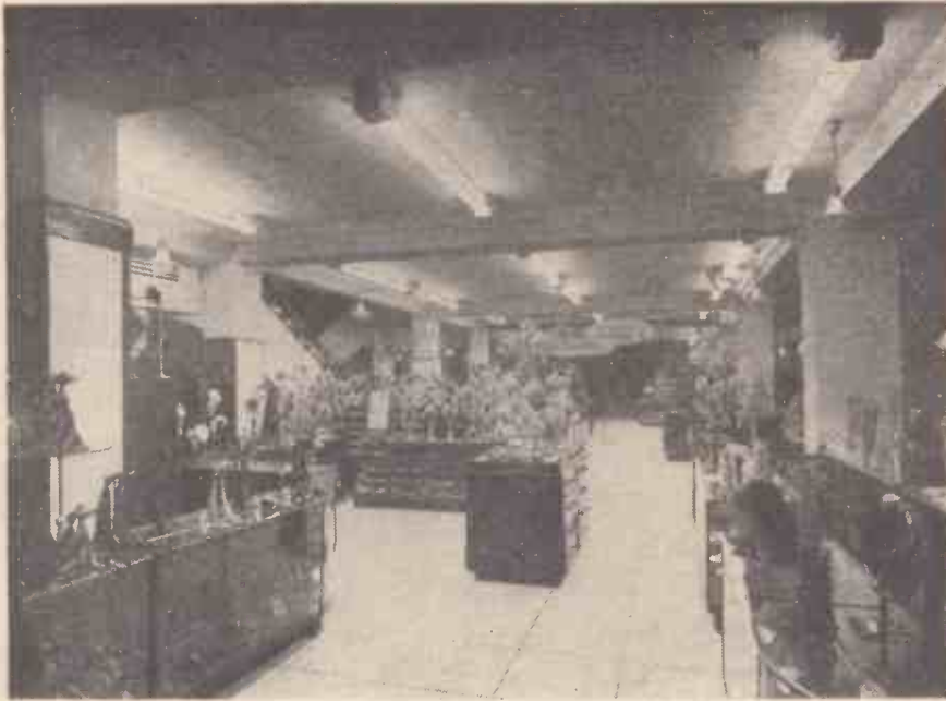
Fig. 3.—G.E.C. fluorescent lighting in a West End store.
