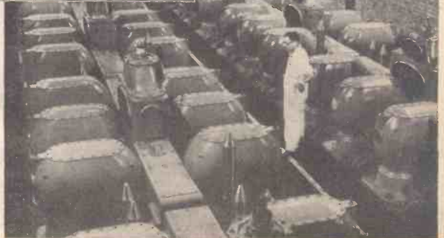
(Above) A corner in the Fulham Power Station showing the feed pumps which supply water to the boilers at the rate of 6,300 gallons per hour per pump.
