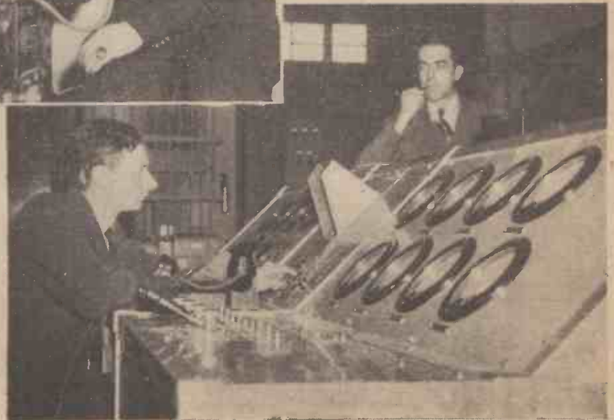
(Below). Mr. J. F. Cartwright at the vision control panel with Mr. Douglas Birkenshaw, the chief engineer.
