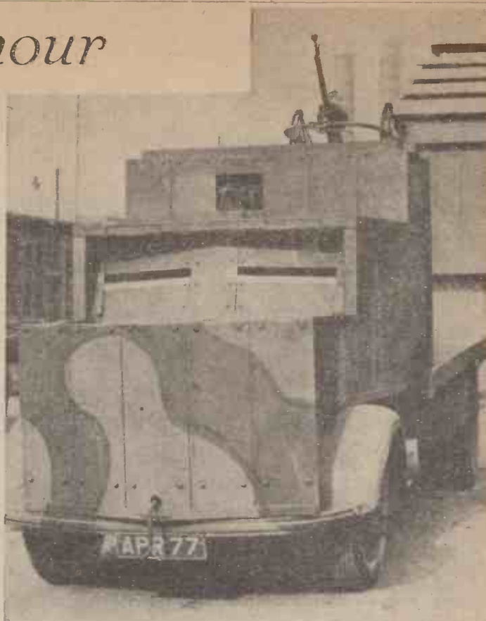
Plastic protective plating on a lorry used for airfield defence.
