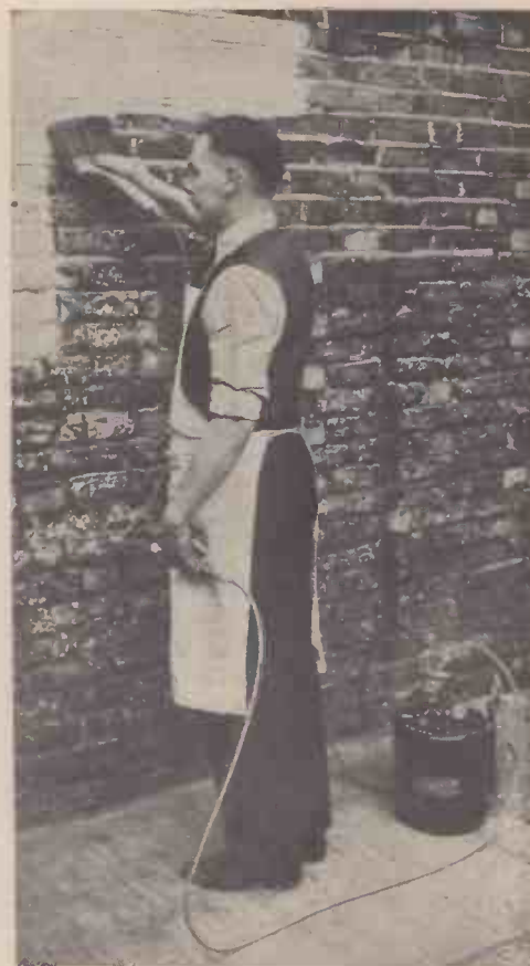
Showing the auto automatic self-feed distemping machine in use, the original photograph of which was taken under practical working conditions.
