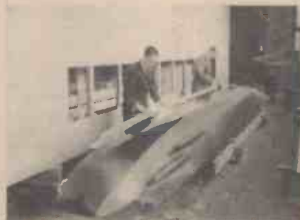
Fig. 2.—Work on the huge hull of the "Queen Elizabeth" at Northampton.
