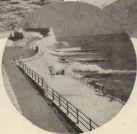
A simple type of seawall at Teignmouth.
