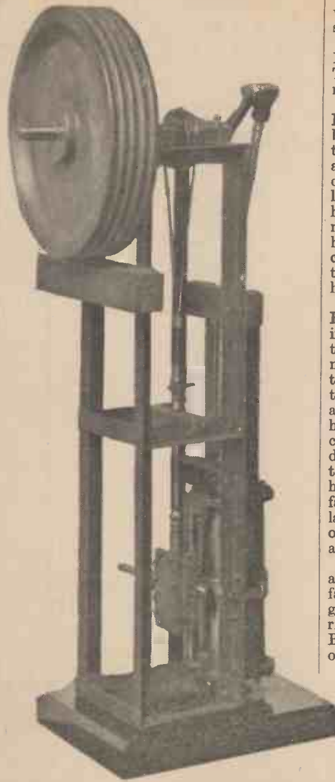
Fig. 3.—The engine of the Henson-Stringfellow model, constructed by John Stringfellow.
