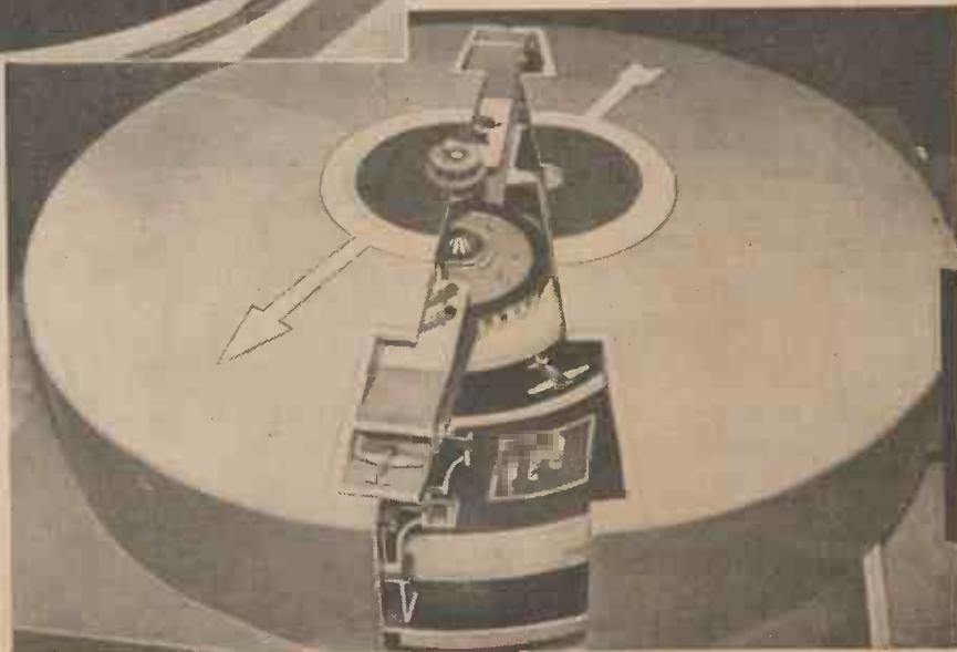
Two interesting photographs of the underground aerodrome showing the internal construction.
