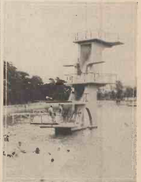
Ferro-concrete is used extensively for diving towers. This fine example at Coate Water (Wilts) is 33 ft. above the surface of the water, which is 10 ft. deep. It cost about £700.
