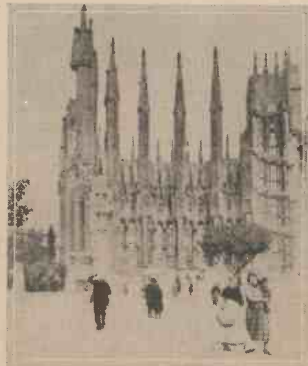
The great new Cathedral at Barcelona—snapped ten years ago when half-finished—showing vertical method of construction.
