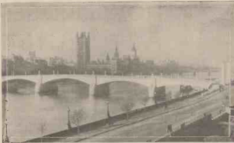
Fig. 21.—Southwark Bridge—a fine example of a reinforced concrete bridge.
