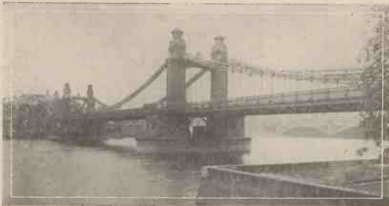
Fig. 19.—A fine view of a suspension bridge. The Chelsea Bridge over the Thames.
