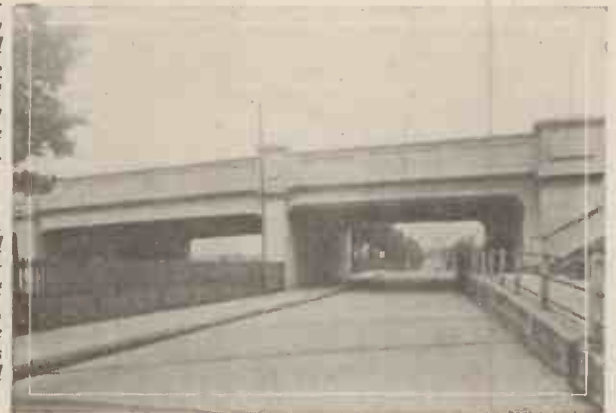
Fig. 14 (left).—An interesting brick-arched bridge with brick abutments that carries a railway over Reigate Road at Epsom.
