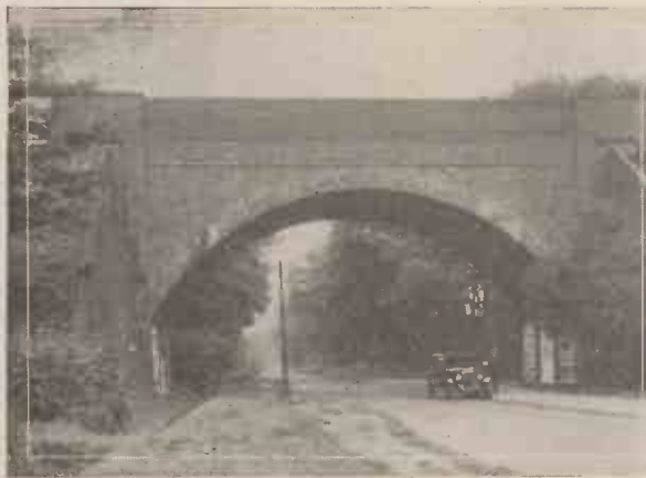
Fig. 14 (left).—An interesting brick-arched bridge with brick abutments that carries a railway over Reigate Road at Epsom.
