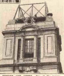
BEFORE AND AFTER. One of the towers of the Alexanira Palace showing the dismantling that taken place in preparation for the erection of a television.mast.
