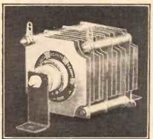
A typical low-tension Westinghouse metal rectifier, suitable for accumulator charging.
