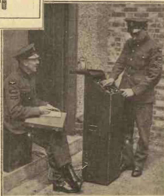
This simple-looking control-box enables the operator to make the "Queen Bee" do just what he wants it to do while it is manoeuvring in the air.
