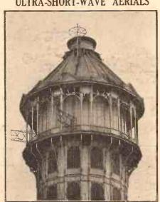
The Baird ultra-short-wave transmitting aerials on the South Tower at the Crystal Palace. The aerials on the balcony are for sound and vision, while that on the top of the Tower is for high-power ultra-short-wave vision transmission.
