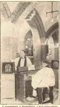
A microphone, a harmonium, a five-valve amplifier and two moving-coil speakers provide the music for St. Margaret's Parish Church, Coventry, since the regular organ broke down. The Vicar considers the tone and volume as good as that of any full-size church organ.
