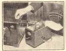
Most Class B units, like the Ferranti one seen here, are extremely easy to add to a receiver. They enable the dry battery user to obtain all the volume he can wish for.
