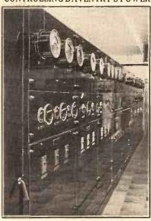
Control of the power to the transmitters at Daventry is effected at this giant switchboard.
