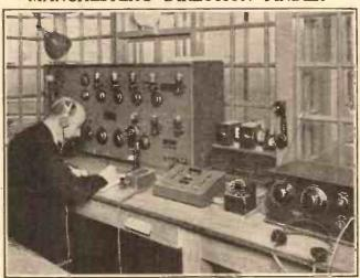
The Manchester municipal airport is equipped with the very latest apparatus for aircraft communication. Here we see the Marconi direction-finding receiver which provides aeroplanes with a ready means of obtaining their bearing.
