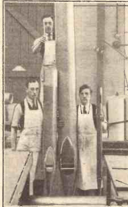
The man at the back is holding a 7" pipe in his hand. The total length of the large central pipe is 18' 6".
