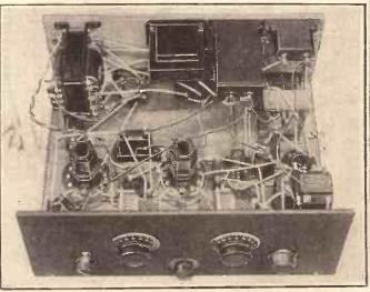
in the mains "mode," the additional smoothing condensers, etc., are placed on an extra "baseboard," at the back.
