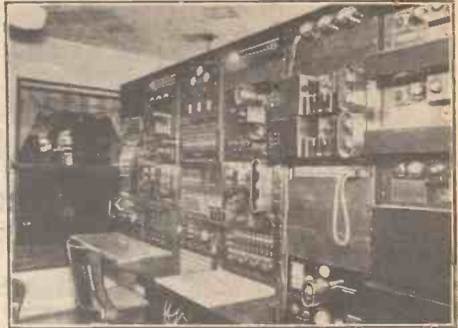
The WCCO control-room at Minneapolis, also placed in a popular hotel. Through this room must pass all the programmes on their way to the transmitter 18 miles away.
