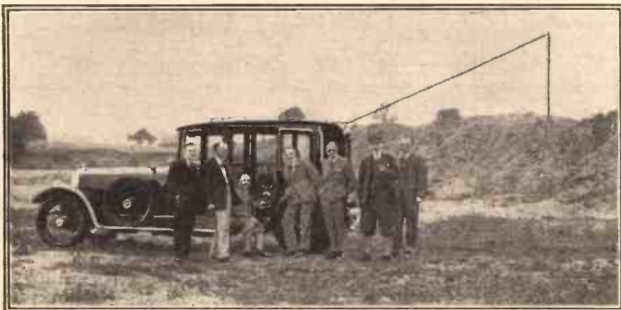
This mobile transmitter belongs to a "go-ahead" North London Radio Society. They are a very enthusiastic group and have done a great deal of very useful experimental work. On the occasion of this photograph they were sending out signals to enable a number of other experimenters with portable direction-finding sets to track them down.
